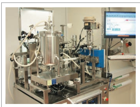
A view of the tangential flow filtration unit situated in the purification process development laboratory.
